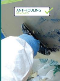
The Poultice Anti-fouling Removal System
